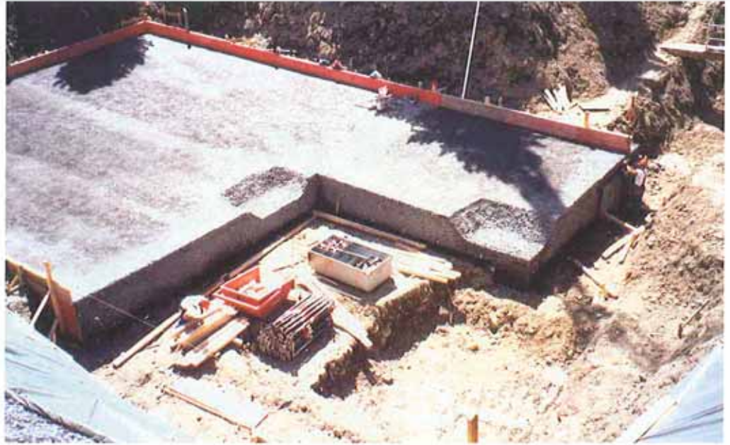
Magerbeton Bodenplatte / Magrone platea
