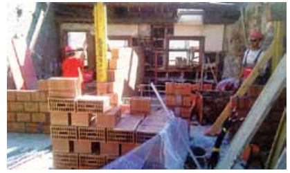
Innenwände in Backstein
