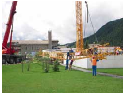
Installation Baukran
